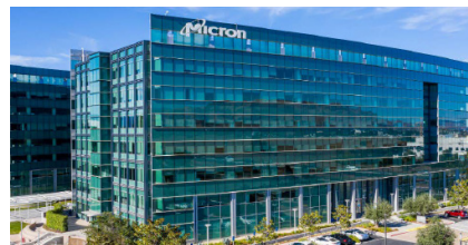
HQ @ First Prime Single Tenant, San Jose, CA
